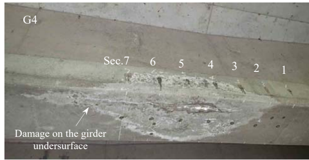
(a) The situation of the crazing (G4).
